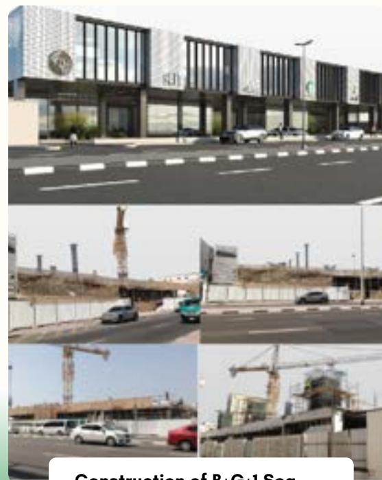
Construction of B+G+1 Sea Mirror Luxury villas - 16
